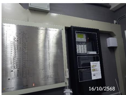
Graphic Annunciator Fire Alarm System
